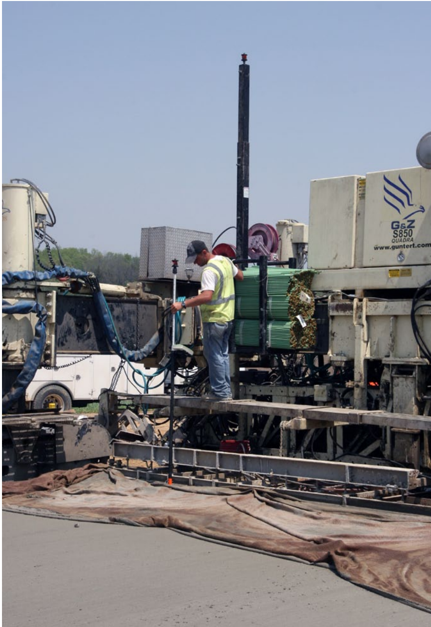
A technician checks the elevation of the fresh concrete slab.
