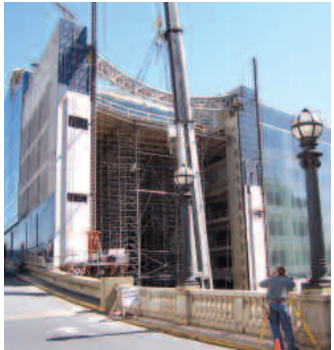
Dax Bird, Midwestern Consulting crew chief, monitors truss installation.
