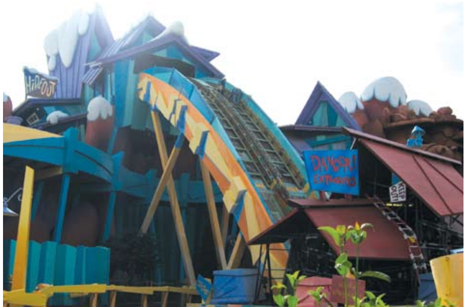
The theme park owner and project contractor specifically requested laser scanning for this project. Image courtesy: JMR Surveying Group, LLC
