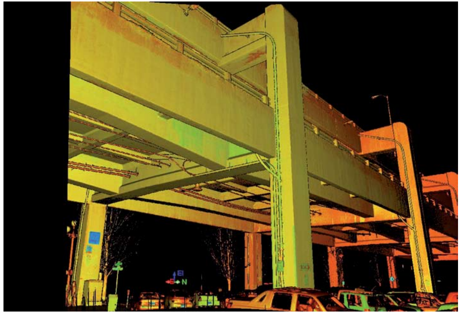
David Evans and Associates keeps three scanners at three different offices. Today, five offices are capable of processing scans into deliverables. Image courtesy: David Evans and Associates
